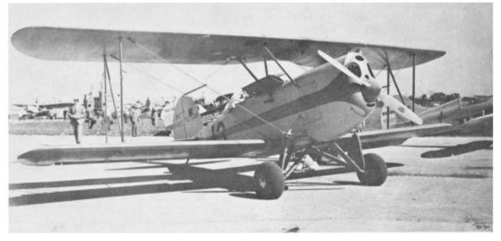
Great Lakes #13. Sandbag ballast and scales for weighing load can be seen on ground aft of left wing.
